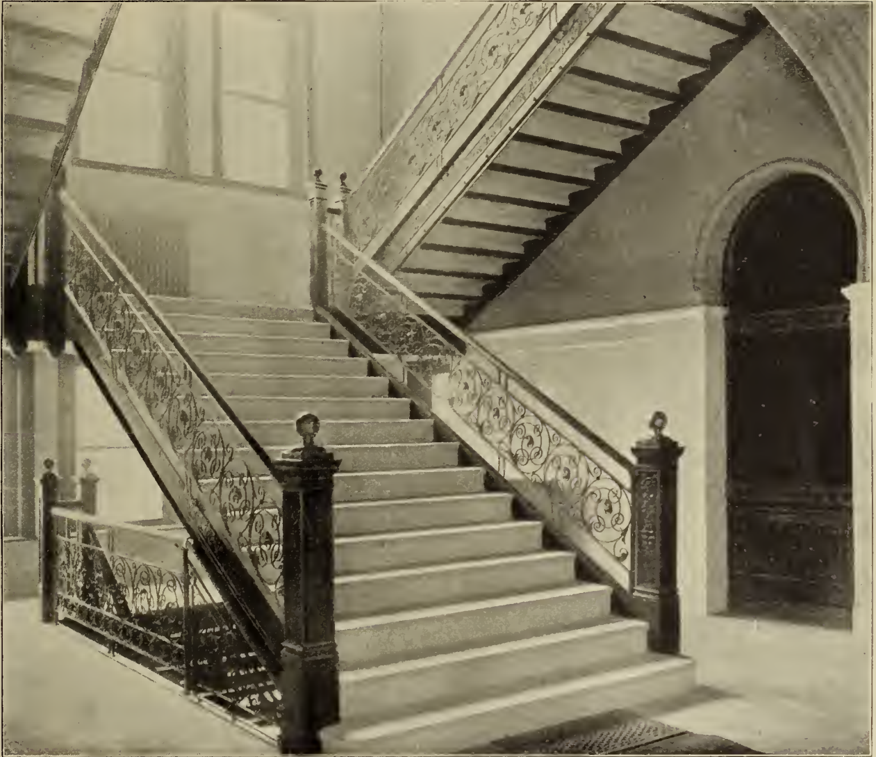
MAIN STAIRWAY, FIRST FLOOR, ARMOUR INSTITUTE, CHICAGO.
